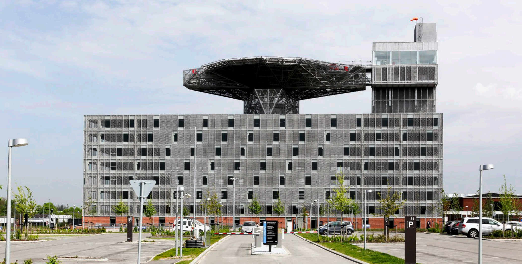
Skejby hospital in Aarhus, Denmark.
